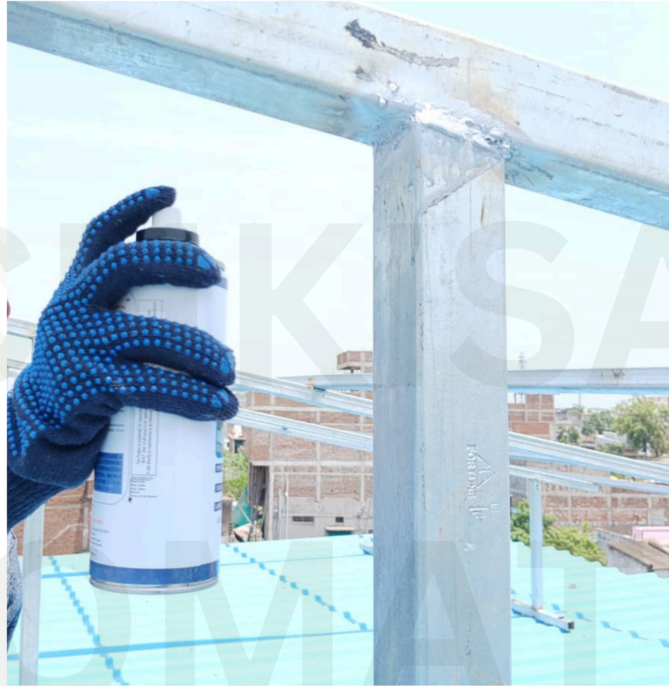
Galvo Spraying to Structure weld
