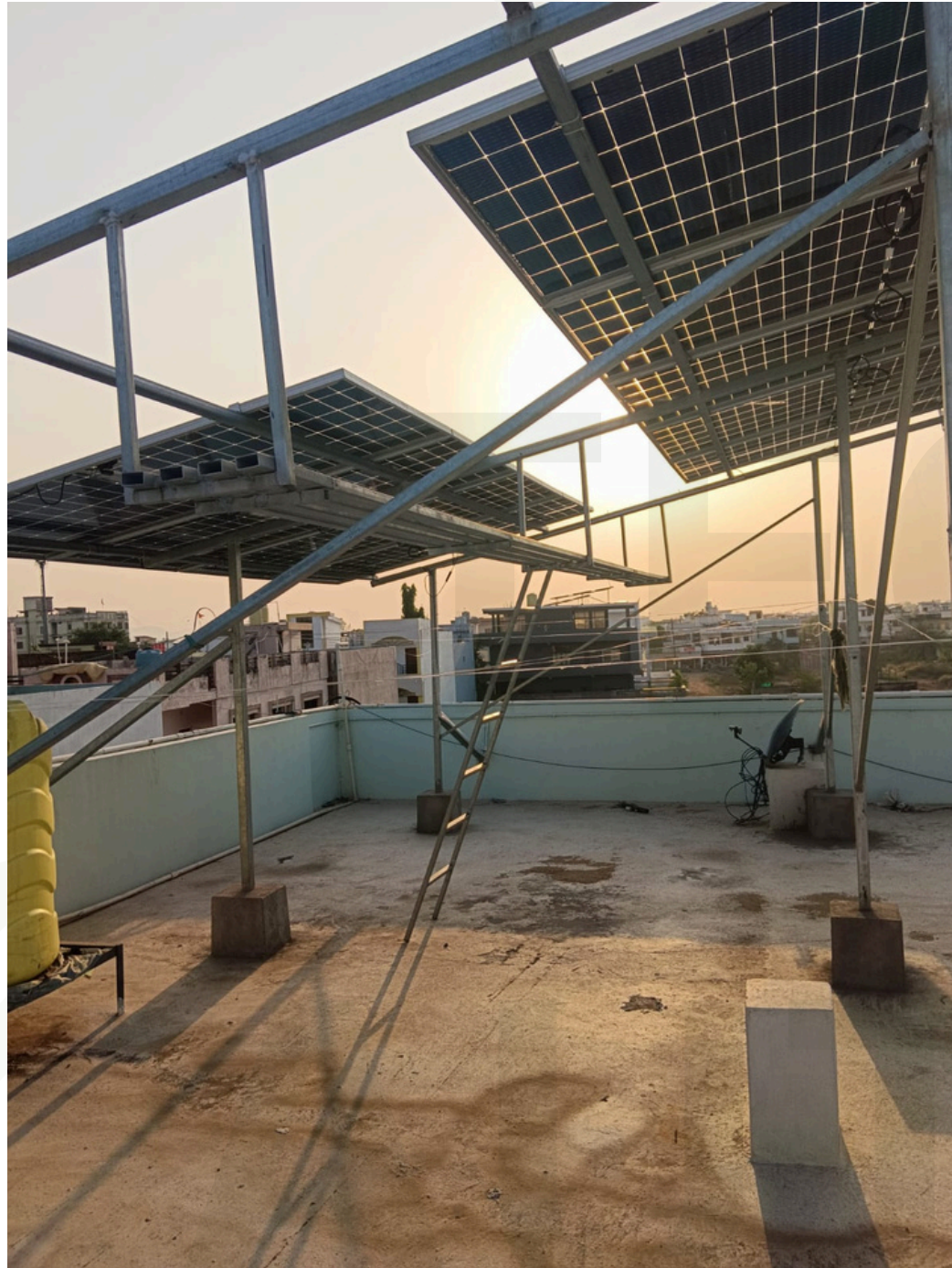
WalkWay in Structure
